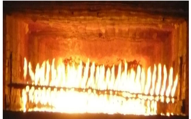
Fig. 6 Ignition vis lances. Tunnel kiln rear view.
